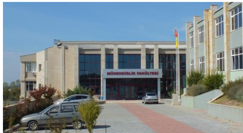
Trakya University Faculty of Engineering Building 3 000 m 2
